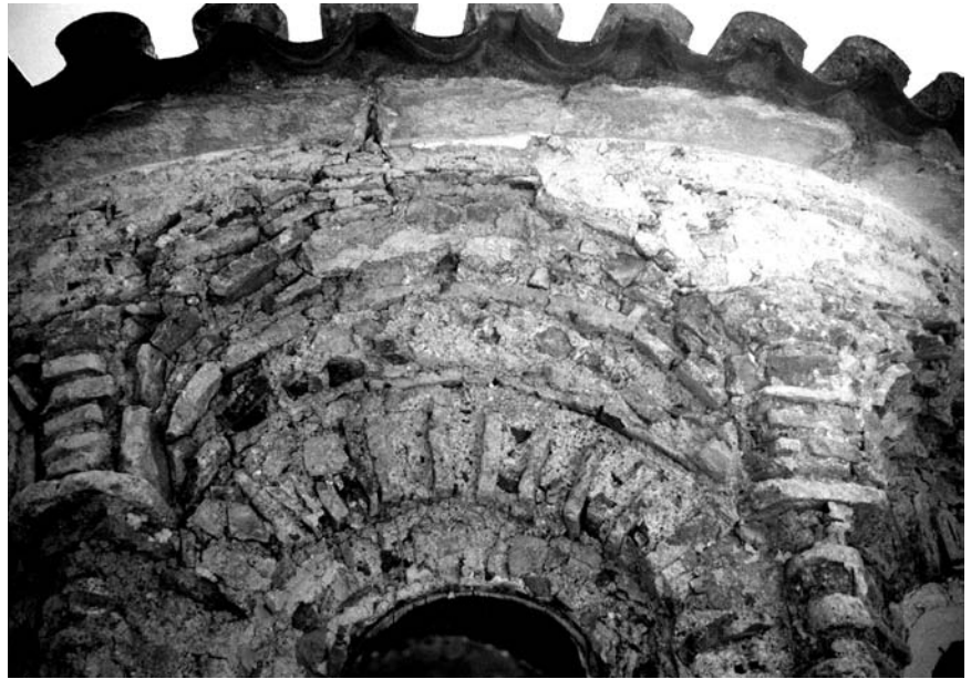
7a) View of the north dome of the exonarthex showing the recessed-brick technique
